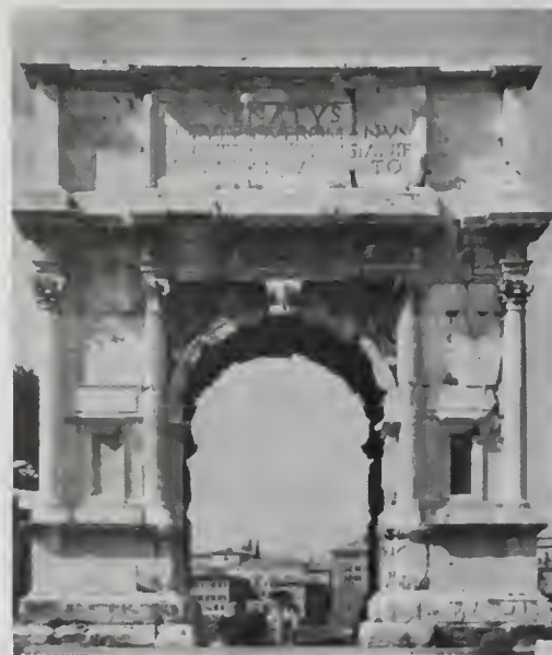
Inscribed attic surmounting the main cornice of the Arch of Titus, Rome, AD 81 A.F. Kersting
